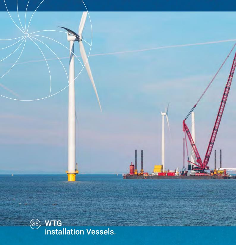
Offshore wind farm WTG installation needs to be done at present using self- elevating barges. However, as the technology improves it might be possible to do this with dynamic positioning heavy lift vessels in the future, as foundations are installed in the present day, to save time and minimise seabed footprints.
